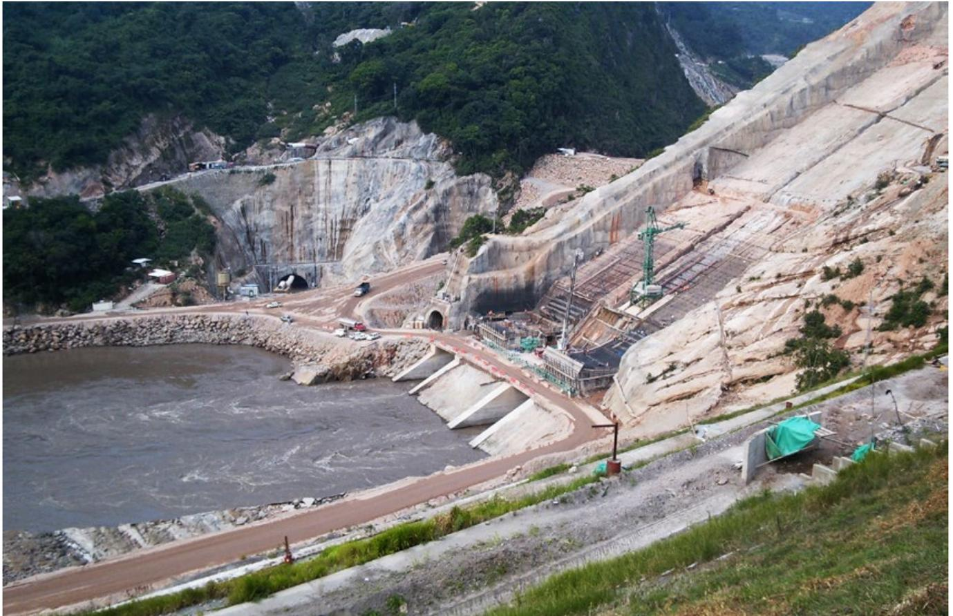
The Sogamoso-Dam is a 190 m high concrete faced rock-fill dam located in northern Columbia on the Sogamoso river. With its installed capacity of 820 megawatts it will increase Columbia's generating capacity by 10 percent. The owner, ISAGEN has awarded JV Company Grupo ICT-II, on which the Company SALINI-IMPREGILO carry out the majority of the civil engineering work.
